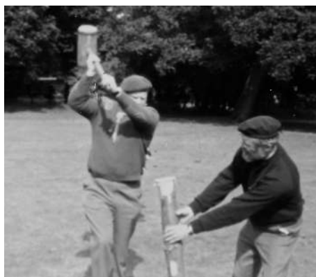
Knocking in pickets for an aerial runway at Whitely Wood Hall 1984
