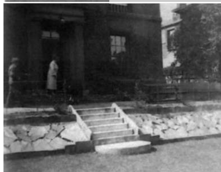
The front door and part of the garden, taken in 1937.
