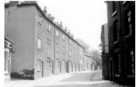
Woodside Lane looking towards Woodfold, demolished in January 1960.
